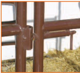
Spring loaded plunger latch
